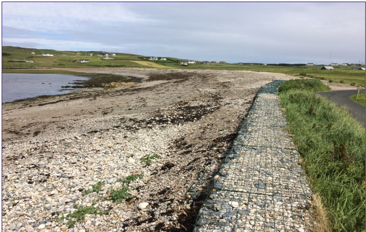
Figure 1.12: Partially buried gabion baskets along the Binbane coast
