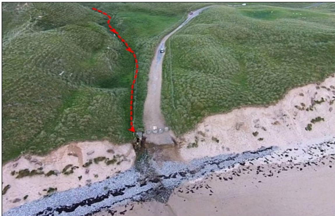
Figure 1.7: Access to Lagg beach on 25 th February 2015 with drainage shown in red (Image: Peter Homer)
